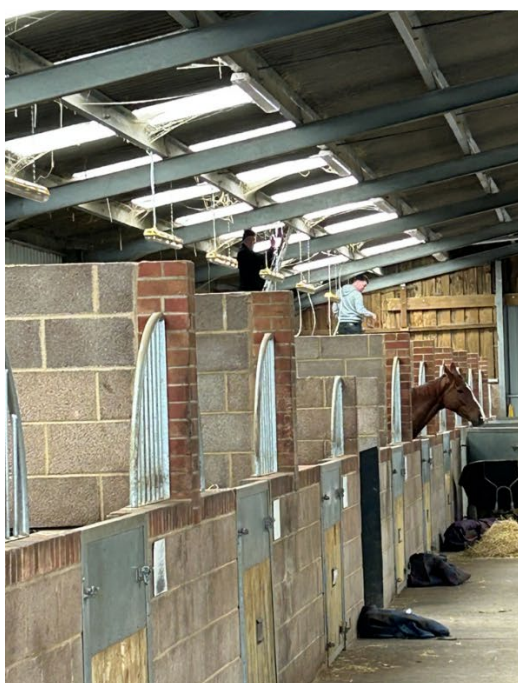
Fig 3: Installation of the Biovitae® technology lighting
